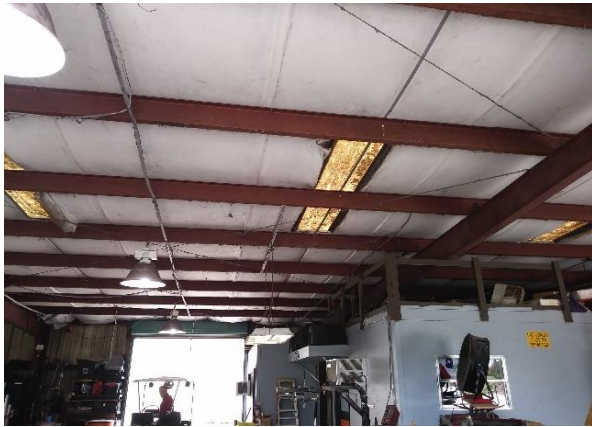
Roof in need of repair in River Run maintenance building.
